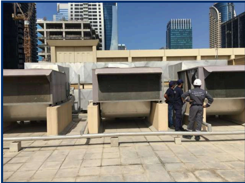
PACKAGE UNIT MAINTENACE WORK- DEWA
