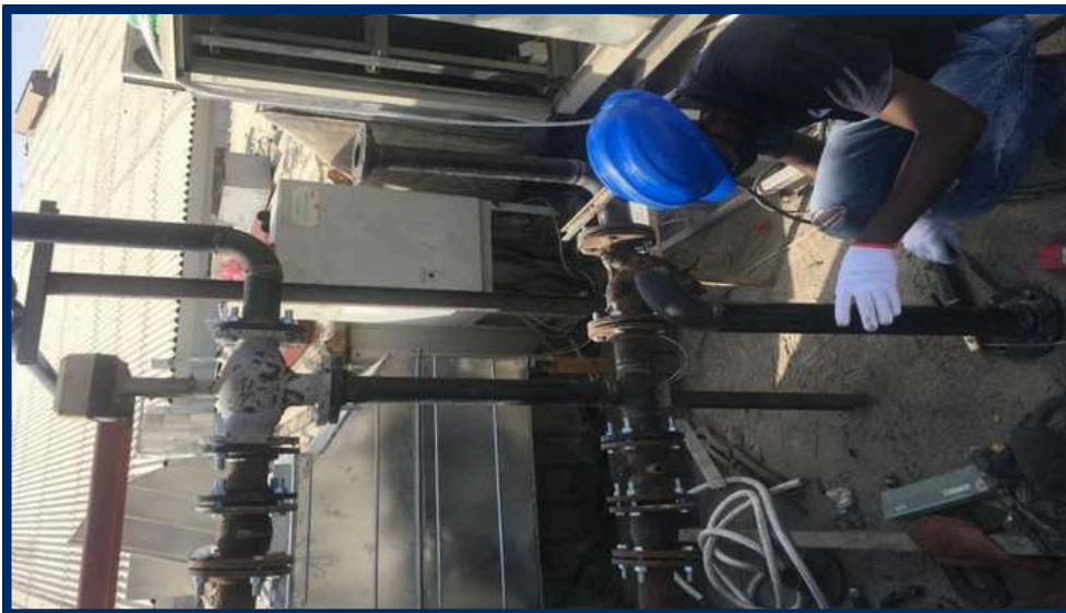
CHILLED WATER PIPING WORK
