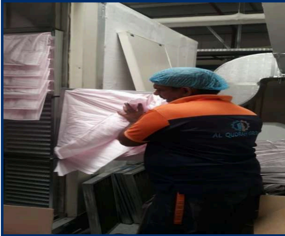
AHU AIR FILTER REPLACEMENT
