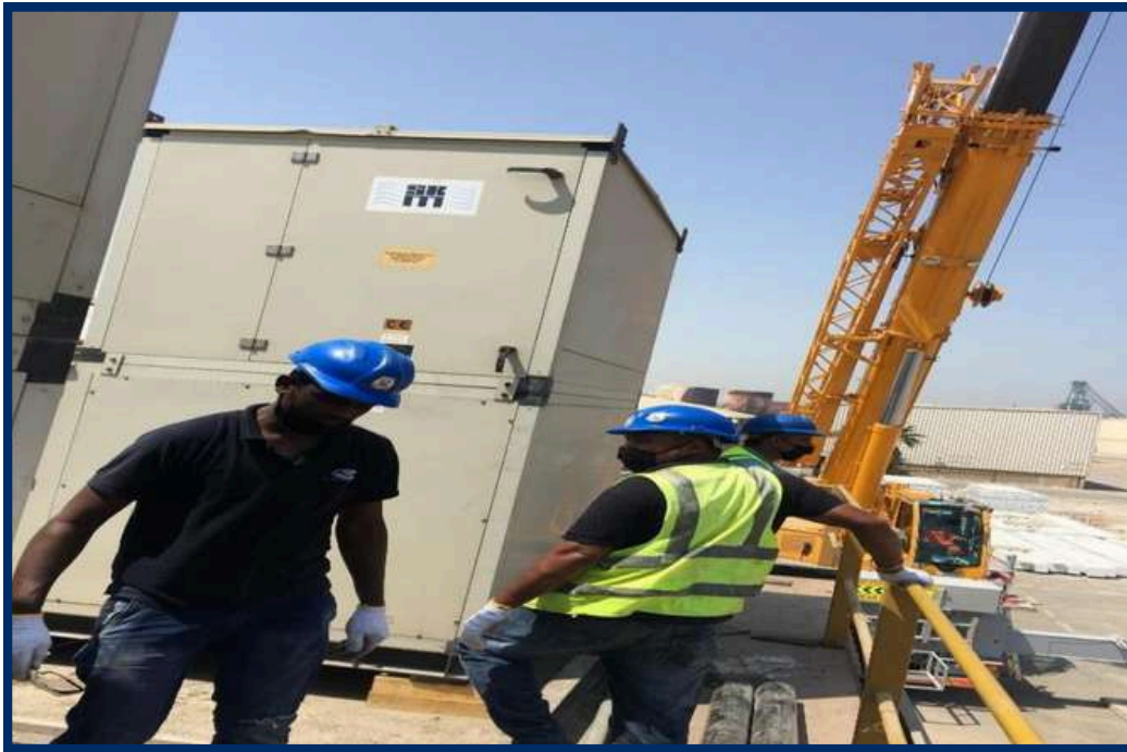
CHILLED WATER AHU INSTALLATION- TIFFANY – KHALID PORT
