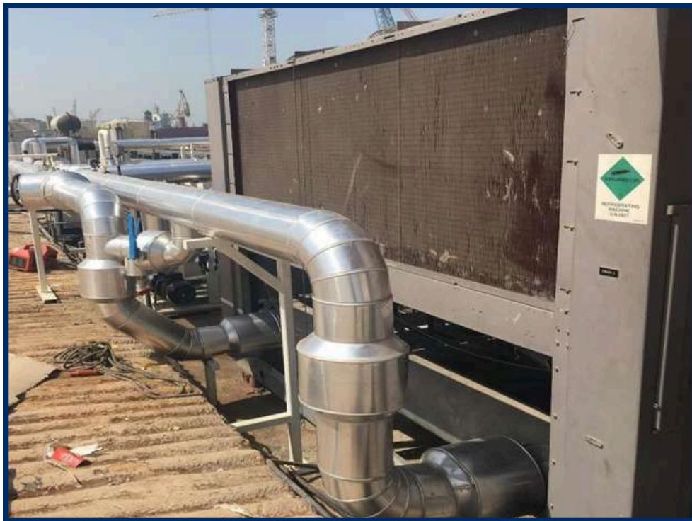
PIPES AND DUCT CLADDING
