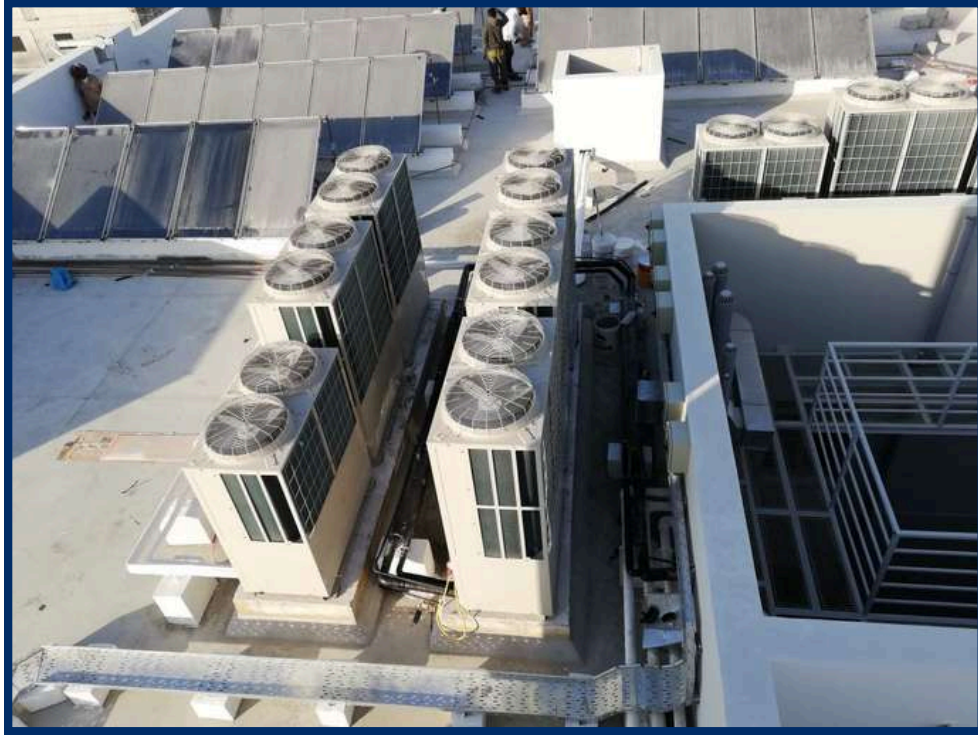
VRV SYSTEM INSTALLATION
