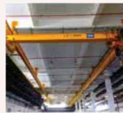
Underslung Crane ( From 100Kg to 15Ton capacity )
