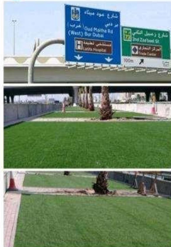
Dubai Municipality Devised road project going on collaborated with Green Scapes at Oud Maitha Road.
