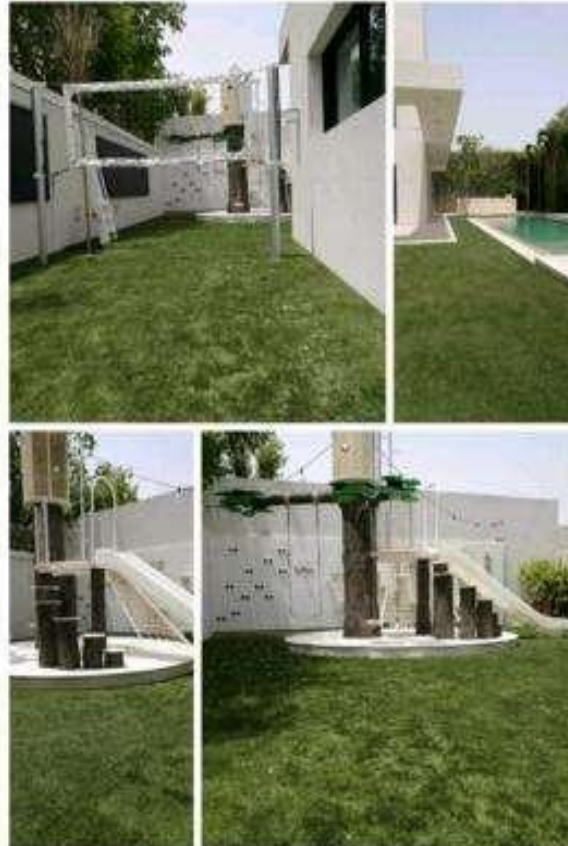
Project for MAGRABI Villa Situated at Jumeirah Handed over on Dated:- 20-Jun-2017
