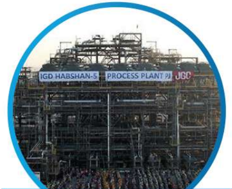
IGD HABSHAN GAS PROCESSING PLANT (GASCO)
