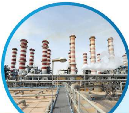
RAS ABU FONTAS DESALINATION PLANT - QATAR
