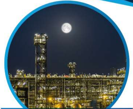
SHA GAS DEVELOPMENT (GASCO)
