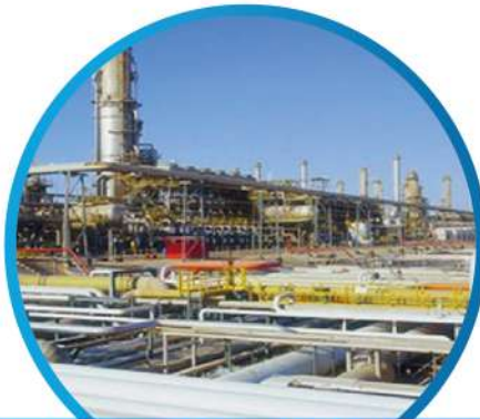
SEA WATER INTAKE PHASE III - RUWAIS (TAKREER)
