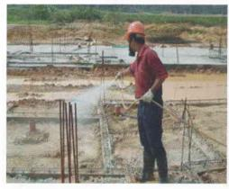
that earth in contact with these surfaces is well treated with the chemical. Before laying the floor, the top surface is also treated with chemicals. We also advise builders to take appropriate care during construction to avoid creating untreated gaps later.
