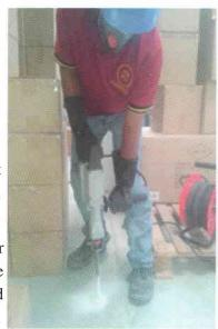
oles will be drilled only along the column side at ground level. If there is loose earth around the walls of the uilding, rodding will be done on every ft. adjacent to the external surfaces of the foundation wall upto a depth f 500 mm from the ground level. If building is surrounded by garden, the treatment shall be carried out to soil, which is in immediate contact with the building.
