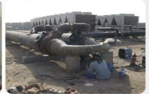
Piping and support work of chilled water plant, ETS Rooms and installation of chillers Heat Exchanger and valves.
