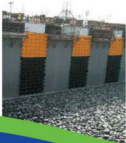
External and internal Stoplogs for Pumping Station at Hamriyah Station for Power Generation & Water Desalination, Sharjah, U.A.E.
