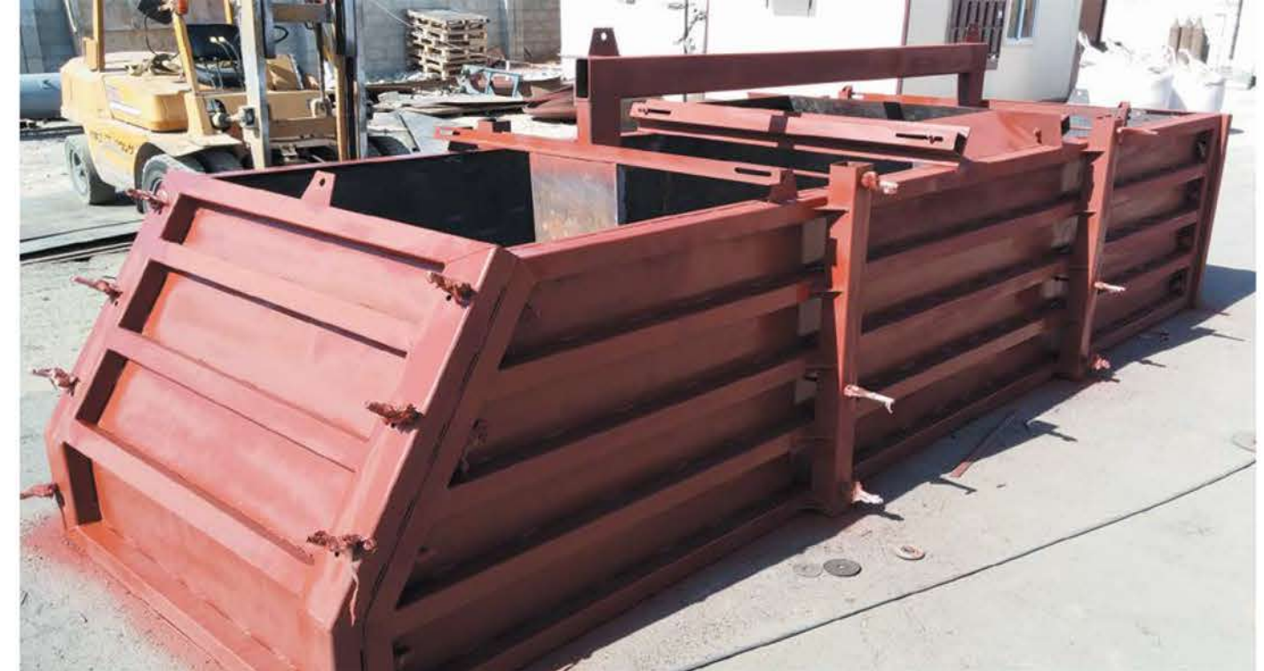
Concrete steel forms - Khalid Lagoon Island Marine Works Sharjah, UAE
