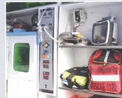
Utility Panel contains O2 flow meters, O2 cylinder changeover switch, central suction control & etc.
