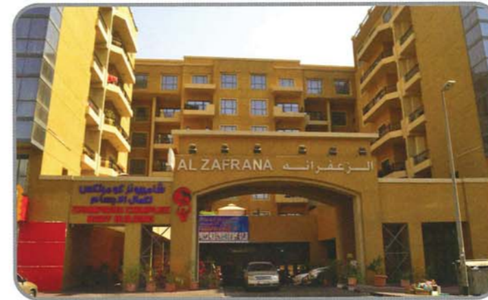
Al Zafrana Res. Building
