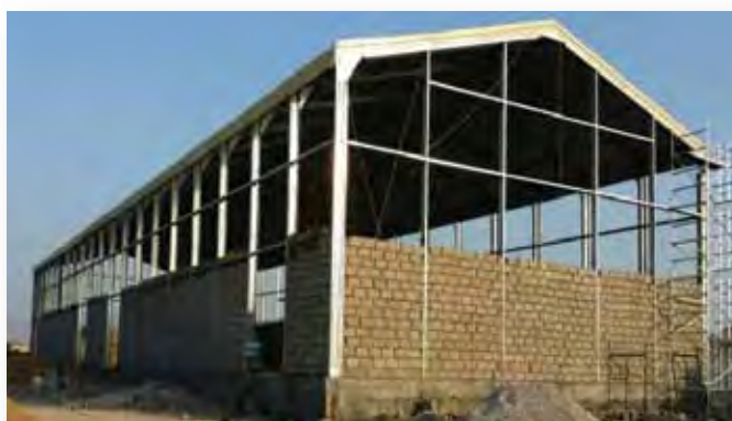
QEB with Concrete Block Walls
