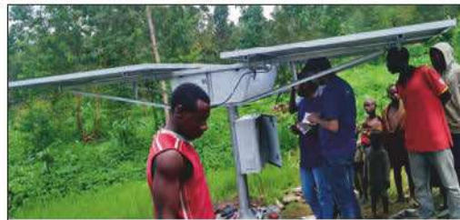
MODEL : 900 WATT, DISCHARGE : 12'000 LPD (WATER & SANITATION CORPORATION, RWANDA)
