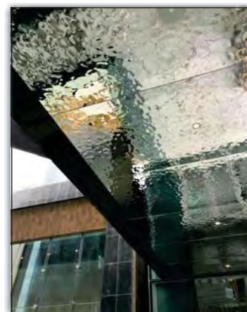
Exterior SS ceiling panel
