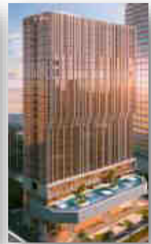
Mama Shelter Hotel (3B+G+24F+R) – 29 Floors in Business Bay
