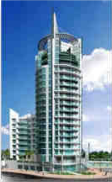
Atlantic Tower (P+G+17F+Gym) - 20 Floors in Marsa
