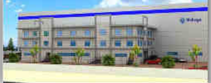
Al Shaya Warehouse in Technopark
