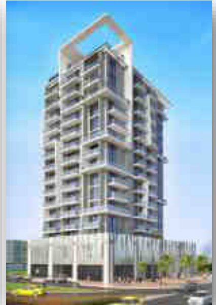
(2B+G+P+13+R) Res. Bldg. - 18 Floors in Al Furjan
