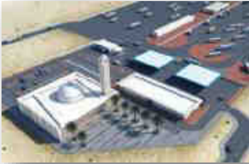
Kizad Truck Plaza Mosque in Kizad, Abu Dhabi
