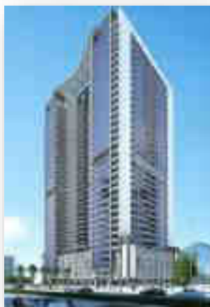
Al Karama Tower (2B+G+4P+31+Gym+R) – 39 Floors in Karama
