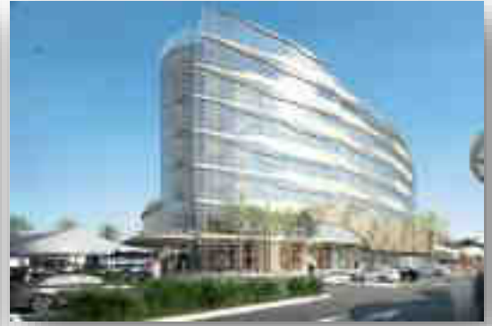
(G+6+R) Danat Al Emarat Hospital Women & Children (South Tower) in Abu Dhabi City
