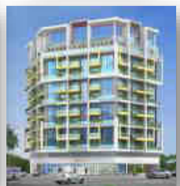
Sunshine Residence Tower (B+G+9Storey+ HC) in DSO
