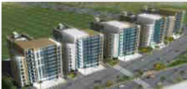
5 Buildings (G+8 Storey+HC) in Dubai Silicon Oasis
