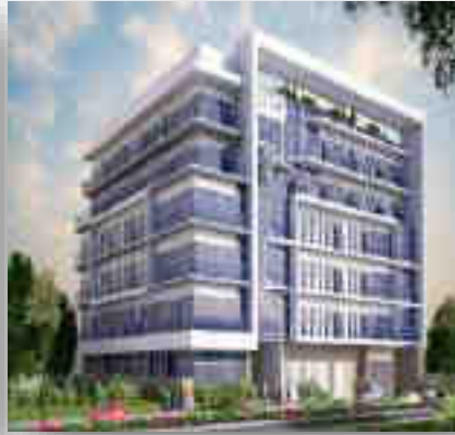
(2B+G+5+Roof) in Jumeirah Village Circle
