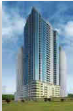
Sahara Tower 4 (G+6P+1/2 Tech. Flr Res. Flr(12th Flrs)+26th Typ+Helipad – 35 Floors in Al Nahda, Sharjah
