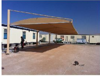
PARKING SHED (CLOTH)
