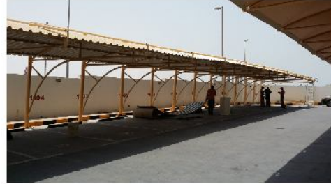
PARKING SHED (SHEET ROOF)
