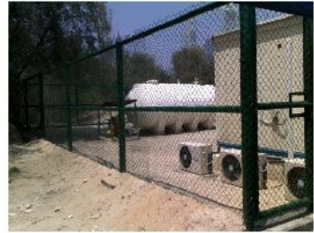
OUT DOOR FENCING
