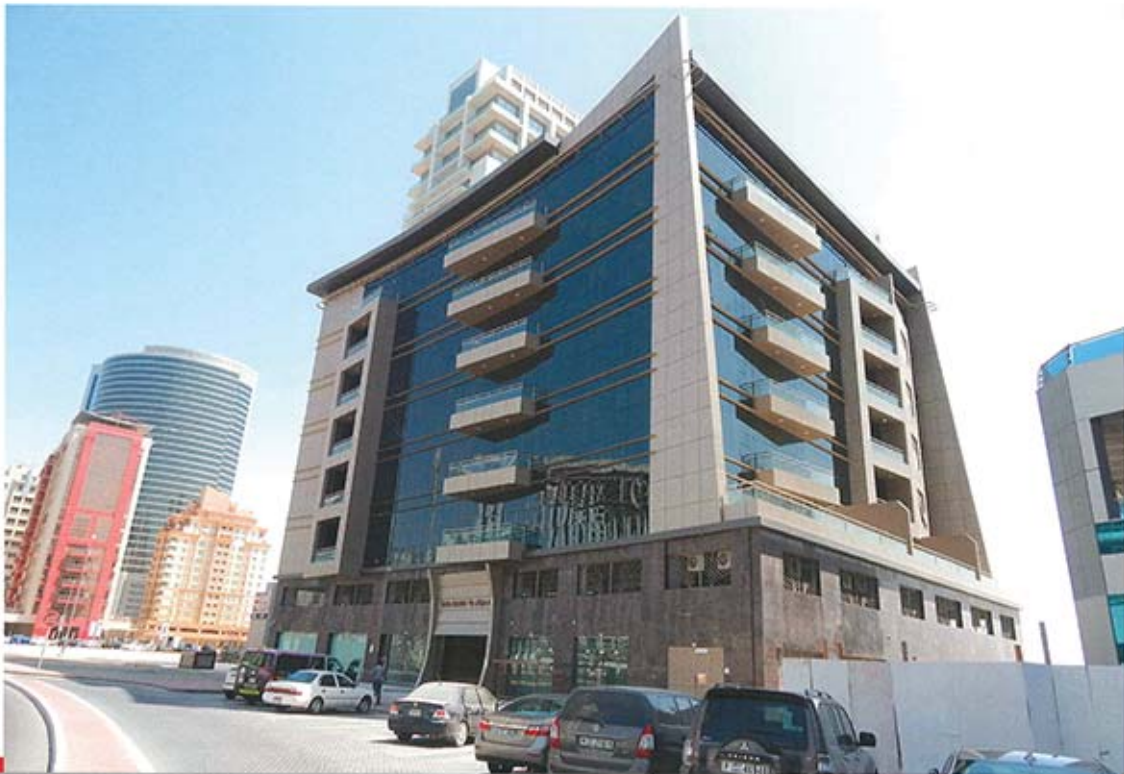
Project: Office Building 4B+G+6+Roof Location: Plot No 373-107, Al Barsha 1 st , Dubai Client: Mr. Ahmad Abdulrahim Ahmad Al Atar
