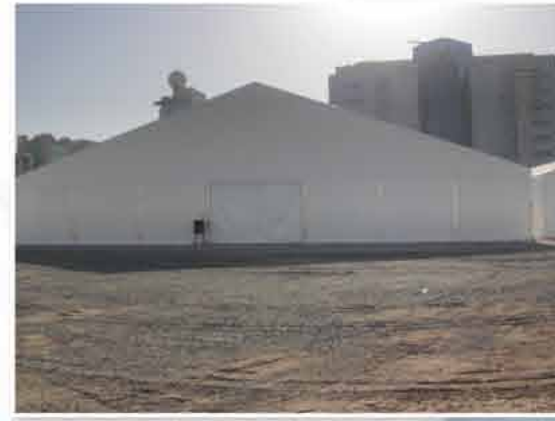
Storage Tent (RT-T06)
