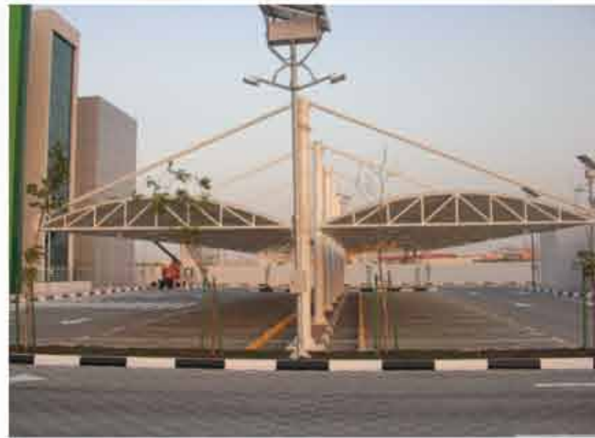
Car Parking Cantiliver Top Support (RT-P02)
