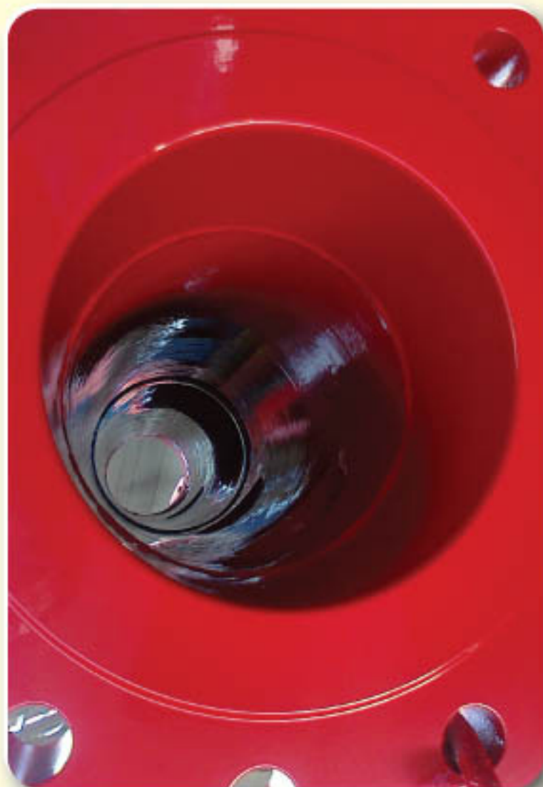
PROJECT: TAKREER OGD PH 111 INTER REFINARY PIPING - FIRE WATER FBE INTERNAL COATING
