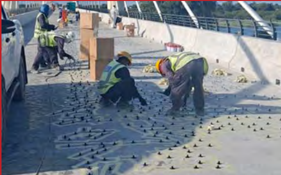
CONCRETE INJECTION, REPAIRS & RESTORATION
