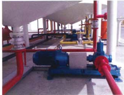
Erection of Storage tanks & Pipe line Fabrication
