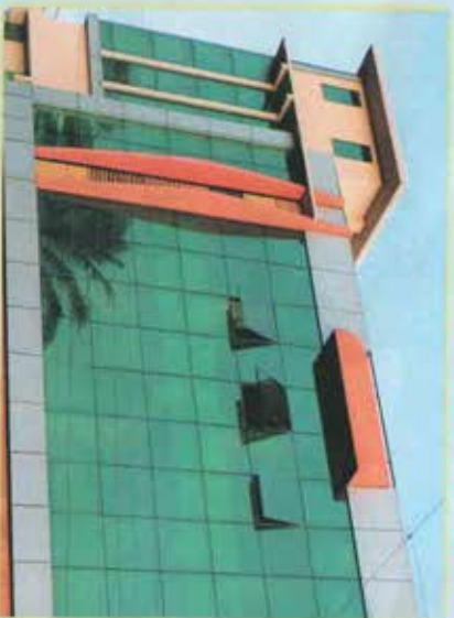
Curtain Wall & Structural Glazing
