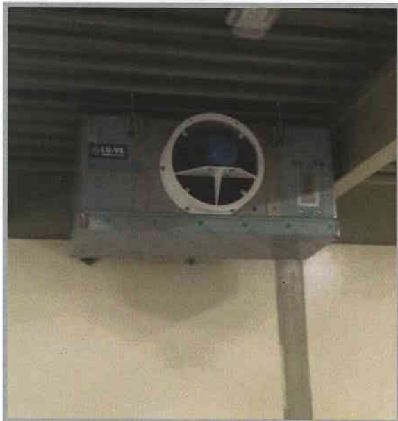
Explosion-proof Motor - ATEX certified
