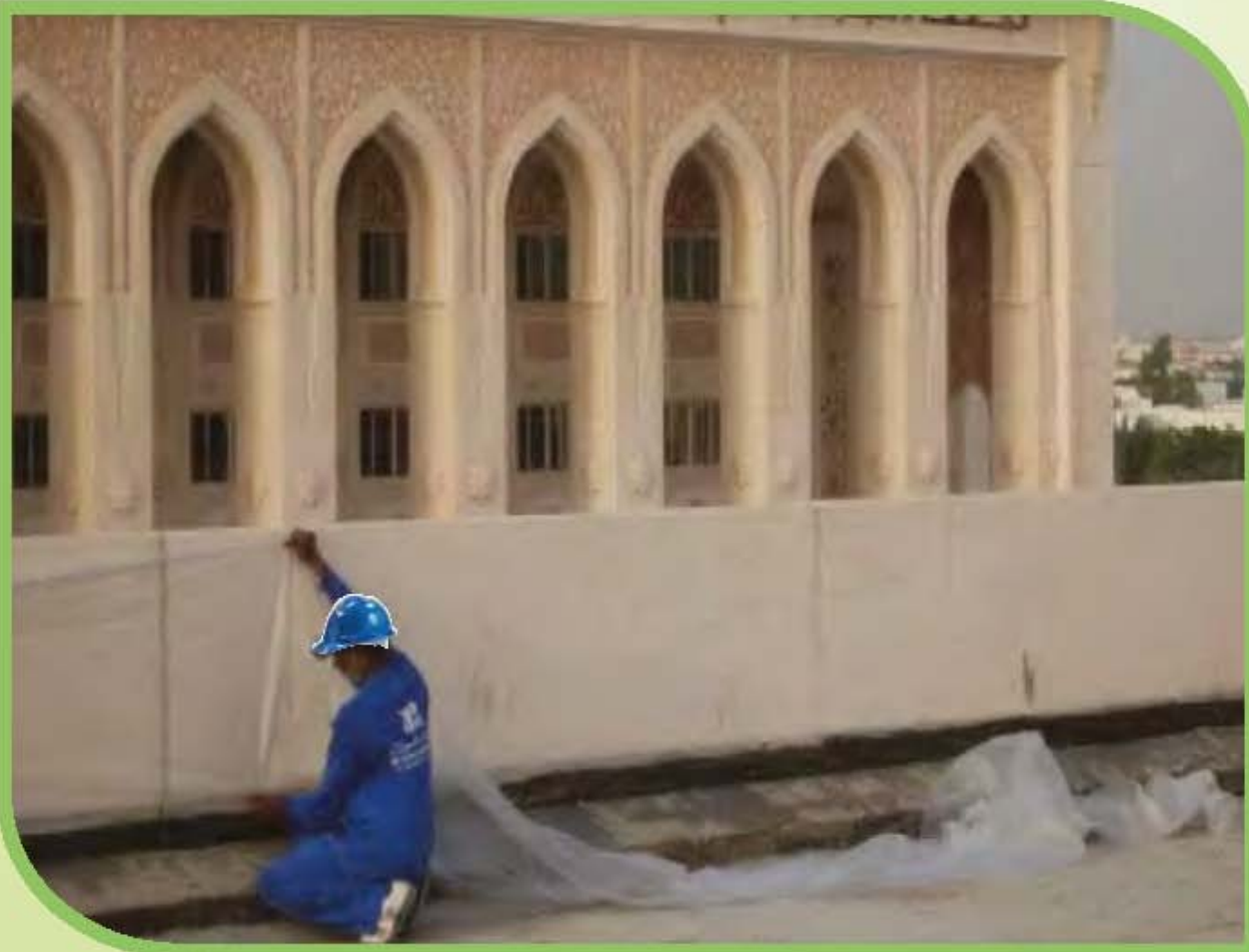
Covering the parapet wall (75 cm height) and other utilities fixed on the roof to avoid the risk of over spray.
