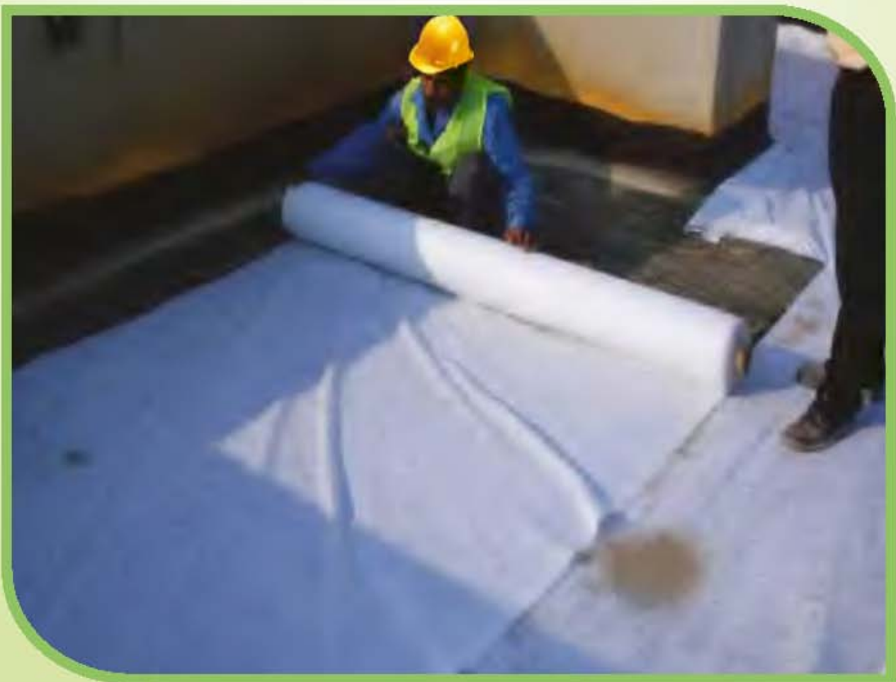
Apply Geotextile Filter Membrane 120 gsm.
