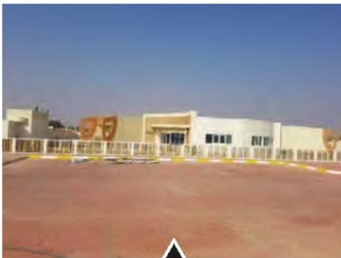
Project: AL FALAH NURSERY Main Contractor: Al Hodoud Building Contracting Co. Consultant: Adnan Saffarini Engineering Consultant. Location: Al Qarren Sharjah.
