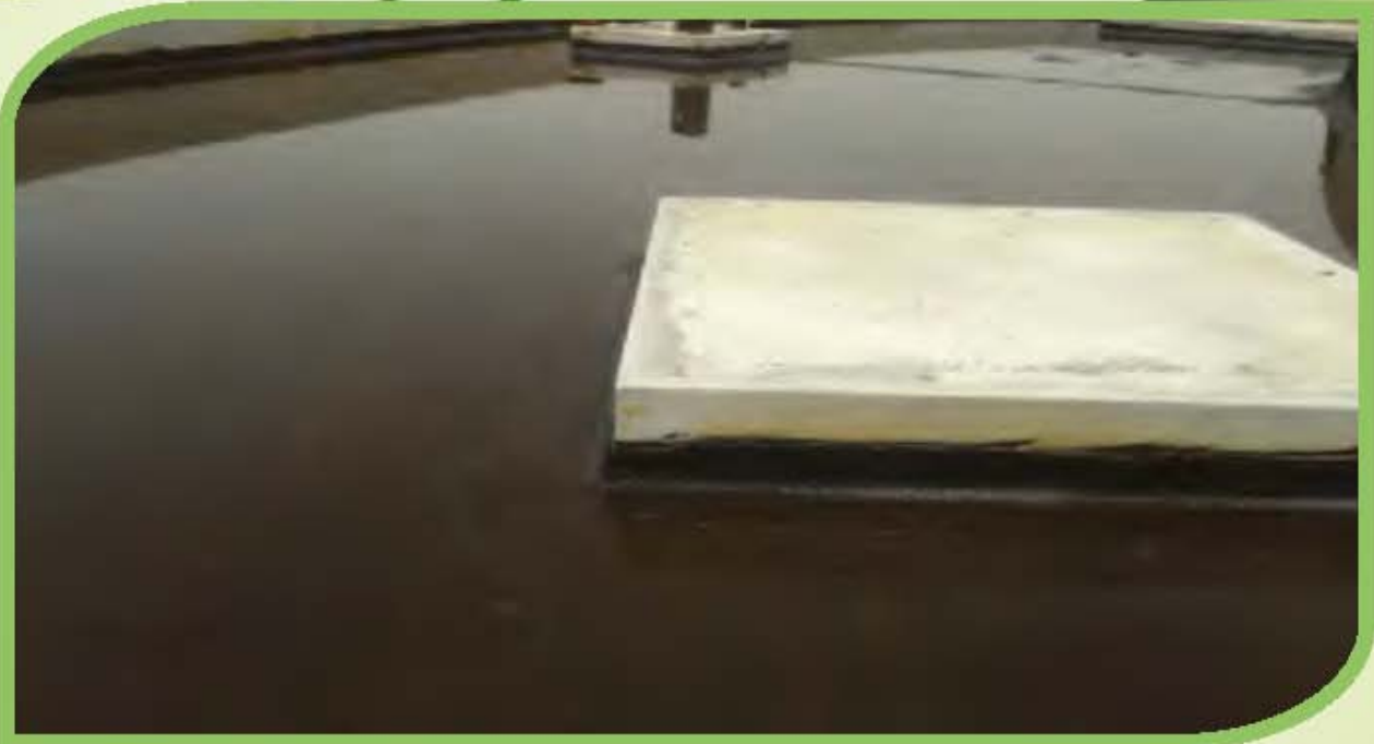
Apply water / leakage test.
