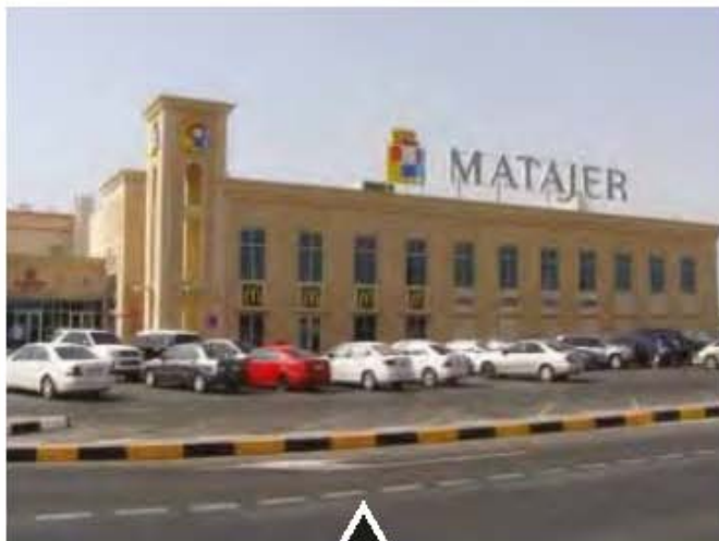
Project: Matajer Mall Location: Al Qous, Sharjah Main Contractor: Habtoor Leightor Group Consultant: Artich Corp Engineering Consultant Type of Works: Combo Roof System
