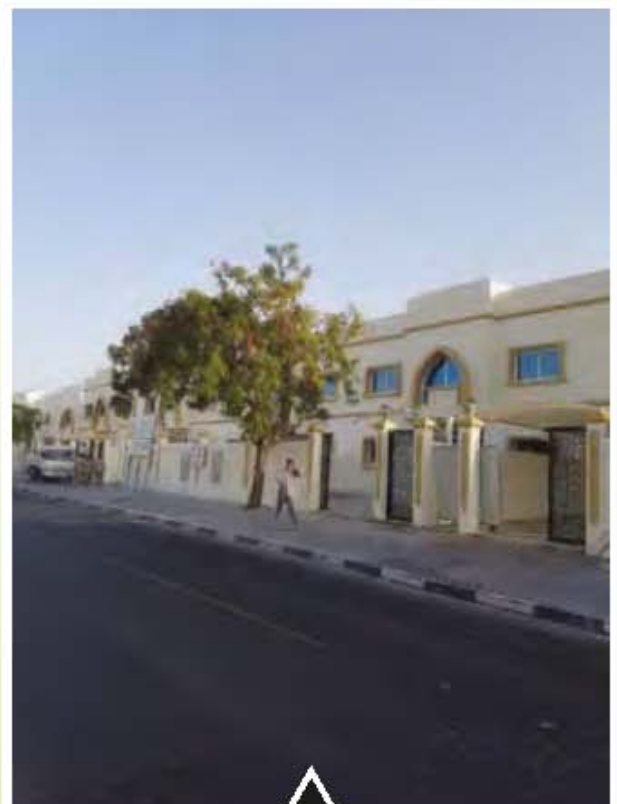
Project: 9 Villas (G+1) For Elsa Bohumad Main Contractor: Solid Contracting Company Consultant: FA Baker Consultant. Location: Abu Hall, Dubai
