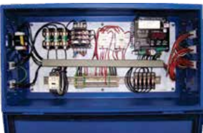
Electrical Control Panel
