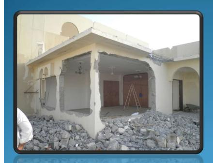
In controlled Demolition we can demolish concrete, block structure according to the site & the situation.
