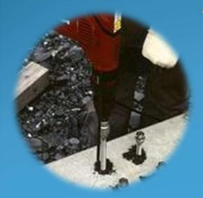
Chemical bolt and anchor fixing is mostly used for hanging steel or increasing steel in columns as well as beams etc. for extensional work.
