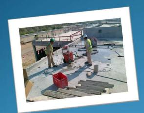
We can cut concrete columns, beams, slabs as well as stairs etc. of different depths using concrete diamond blades. With Concrete Saw Cutter, we cut concrete up to the limited depth. This machine is operated through remote control and having a wide range of safety system.
