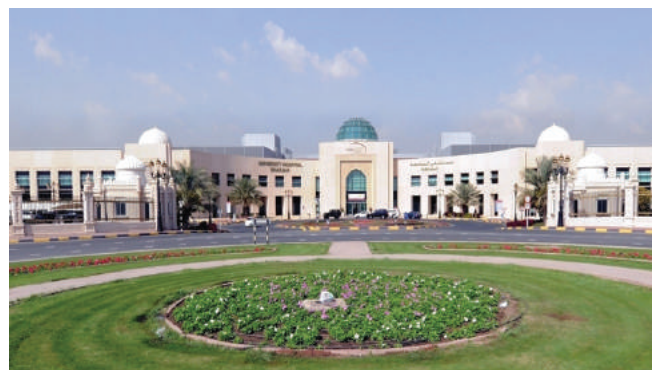
University Hospital Complex, Sharjah, UAE
