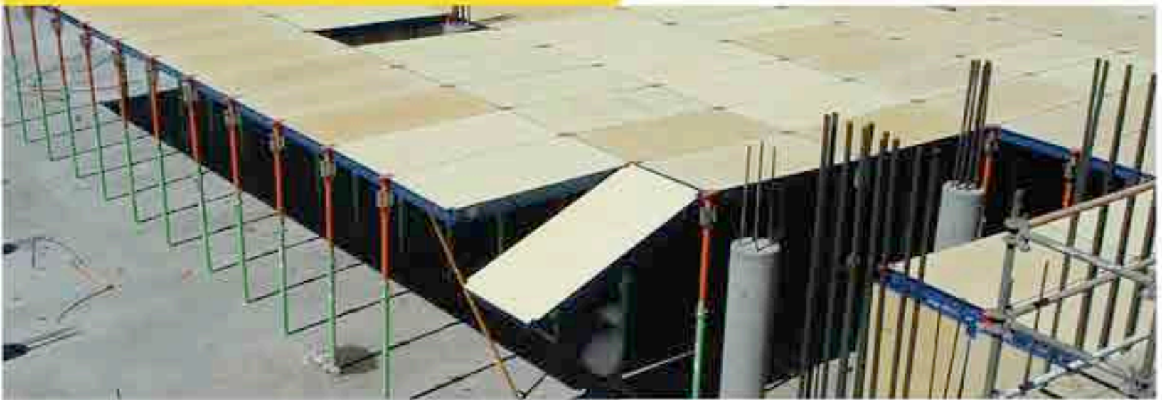
Panels, Props and ADT in use at a construction site in Washington.
