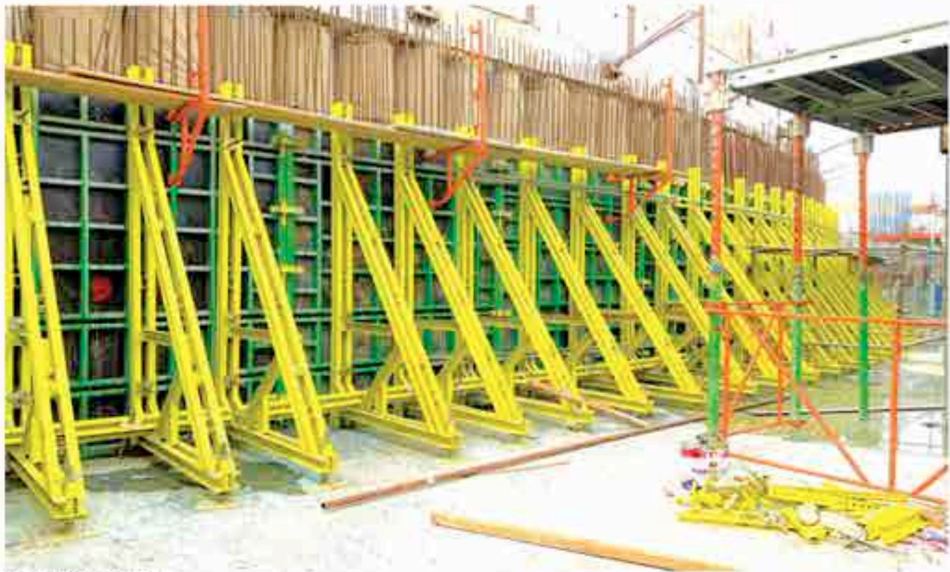
TB1 Retaining Wall
