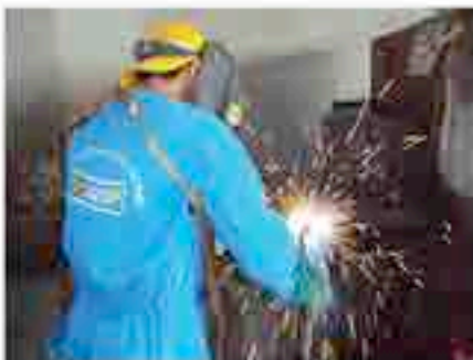
Welding and Fabrication Facility
