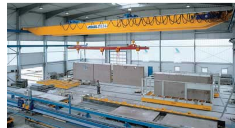
ABUS ZLK double-girder travelling crane with two tandem-controlled electric wire rope hoists and a spreader used for carrying prefabricated building components (Raab).
