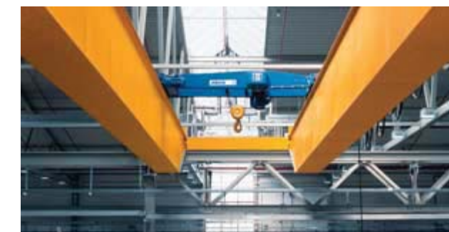
This installation benefits from the ultra low headroom design of the ABUS type DQA wire rope hoist (Bien-Haus).
