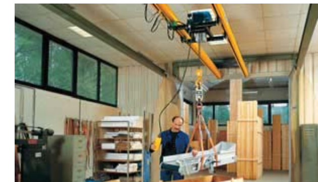
This ABUS ZSB double-rail system makes it easier to lift bulky items into crates (MTF Technik).
