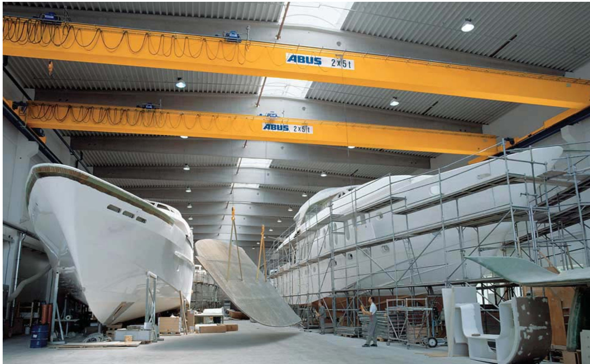
ABUS ELS single-girder travelling cranes with two wire rope hoists used for handling superstructure components for luxury yachts (PR Marine Boatyard)
