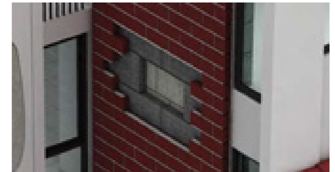
Cavity Wall Insulation Suggested Product: STYRO Graypor 180
