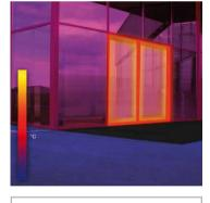
Modern building frontages, let down only by entrances with conventional, non-thermally-insulated profiles = unnecessary loss of energy.
