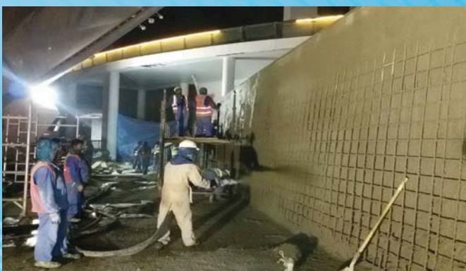
The lower wall was sprayed with gunite to a thickness of between 10cm to 25cm to form an inclined slope and strengthen the wall
