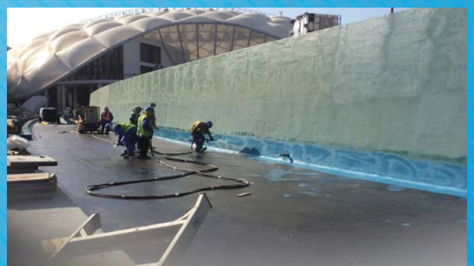
Water proof membrane being sprayed carefully to the floors and walls of the fountain pools
