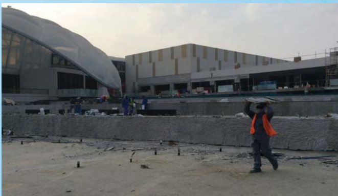
All the granite tiles and coping were removed including existing water proof membrane
